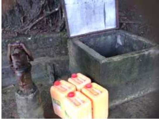
Figure 1. Barangay 13 Diversion Road Deep Well
