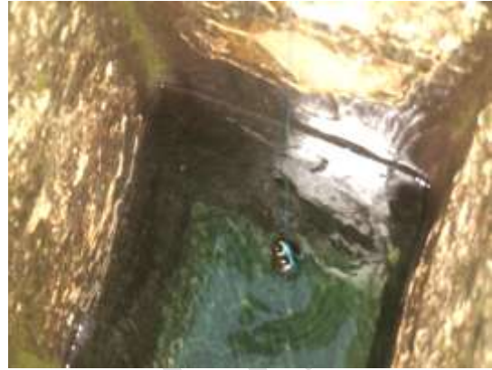
Figure 2. Barangay 7 Deep Well
